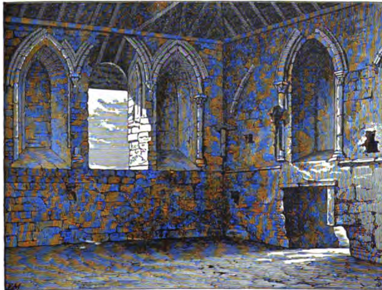
INTERNAL VIEW OF THE WEST END OF HARDHAM PRIORY CHAPEL.
